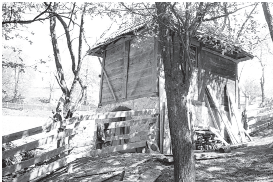
Image 22. A vajat with a frame and an infill of horizontal planks standing on a dressed stone basement
