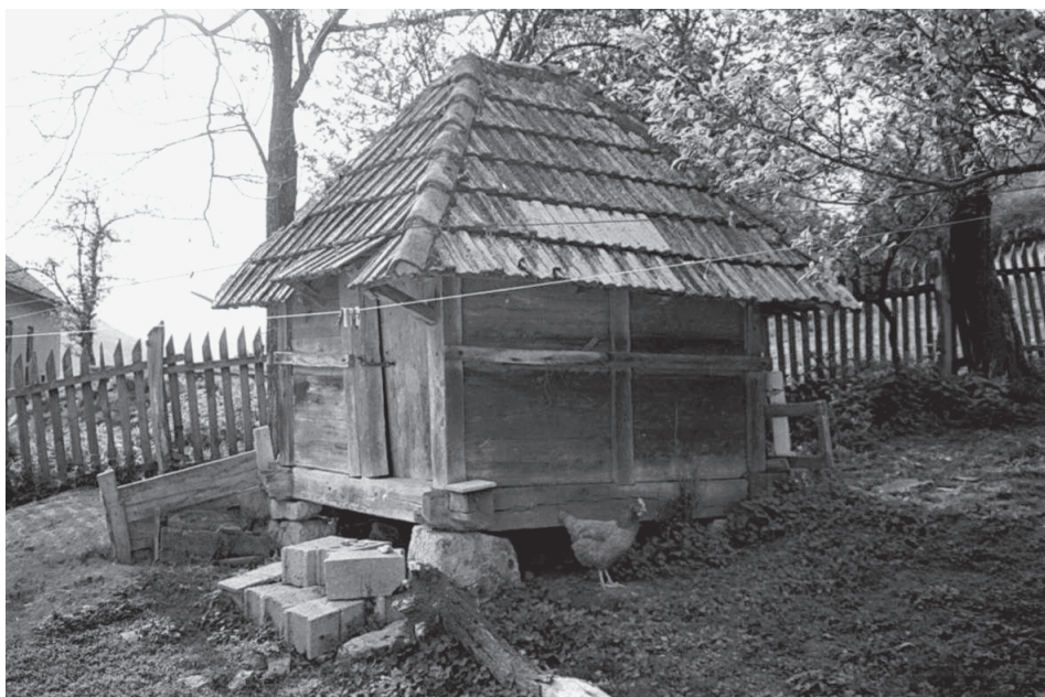
Image 10. A vajat with a frame and an infill of horizontal planks
