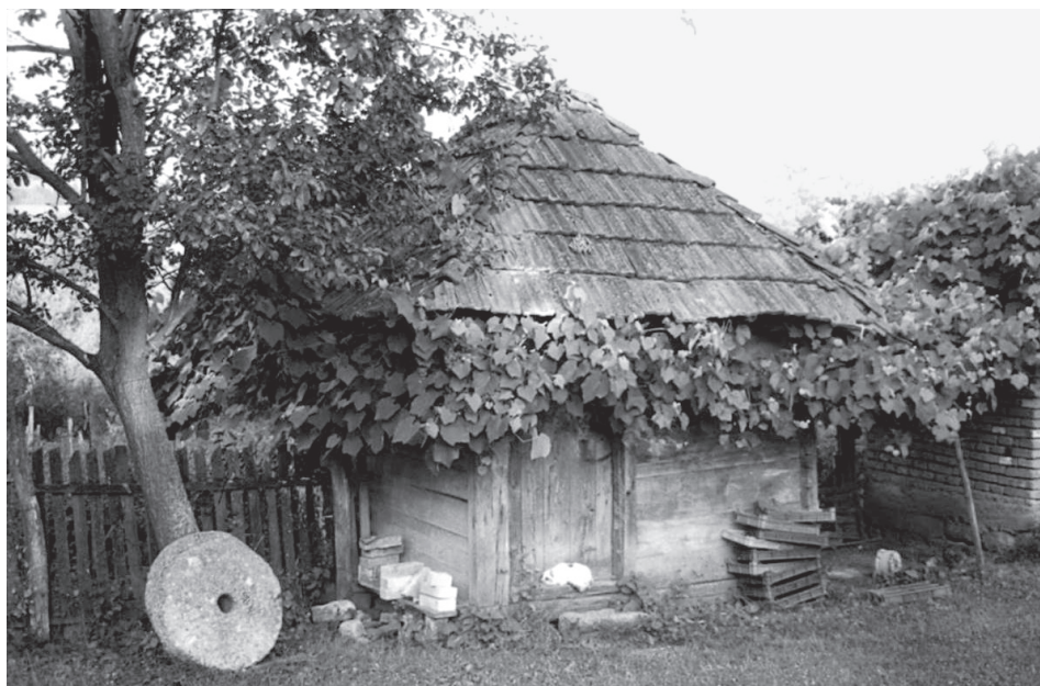
Image 12. A vajat with a frame and an infill of horizontal planks
