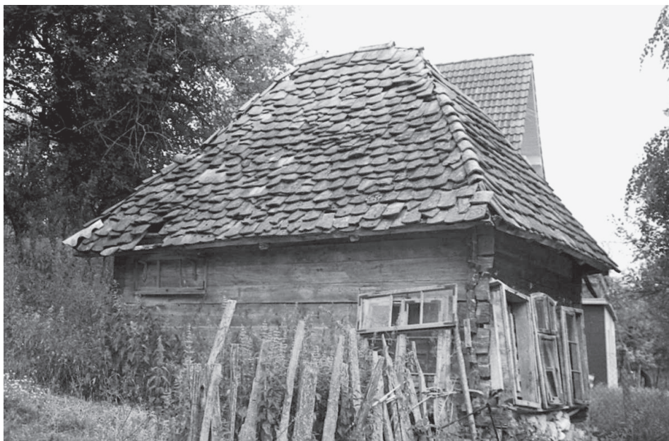
Image 4. A vajat made from thick planks which are connected with halving joints
