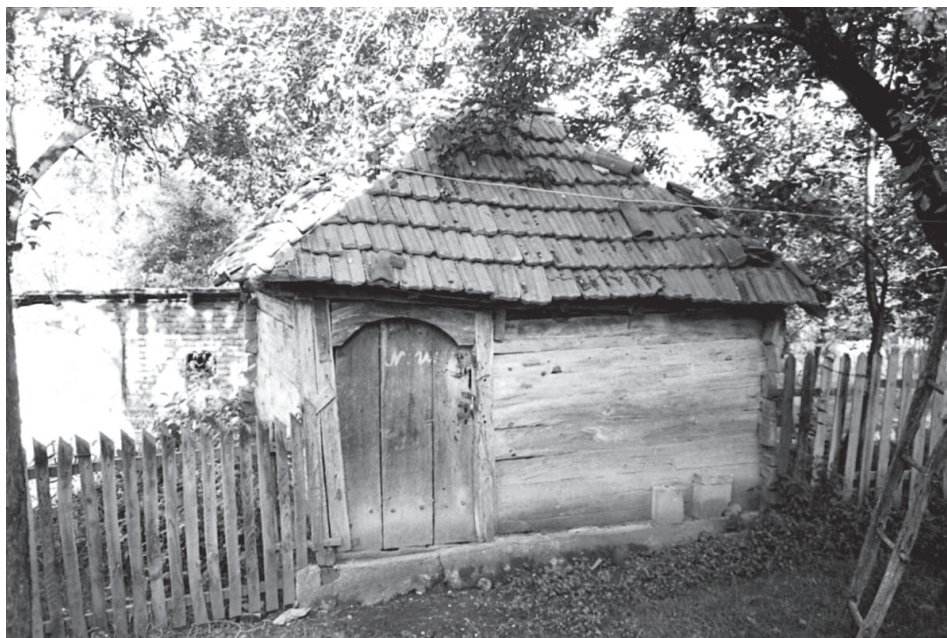
Image 5. A vajat made from thick planks which are connected with halving joints
