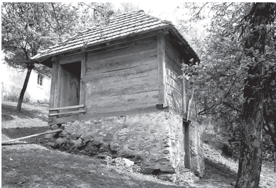
Image 21. A vajat with a frame and an infill of horizontal planks standing on a dressed stone basement
