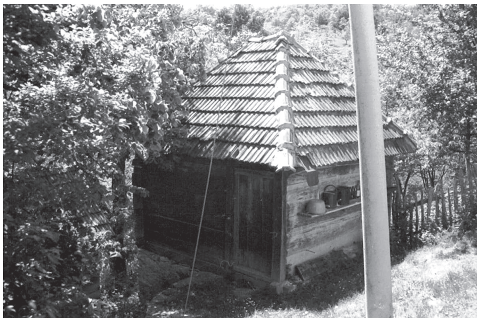
Image 6. A vajat made from thick planks which are connected with halving joints
