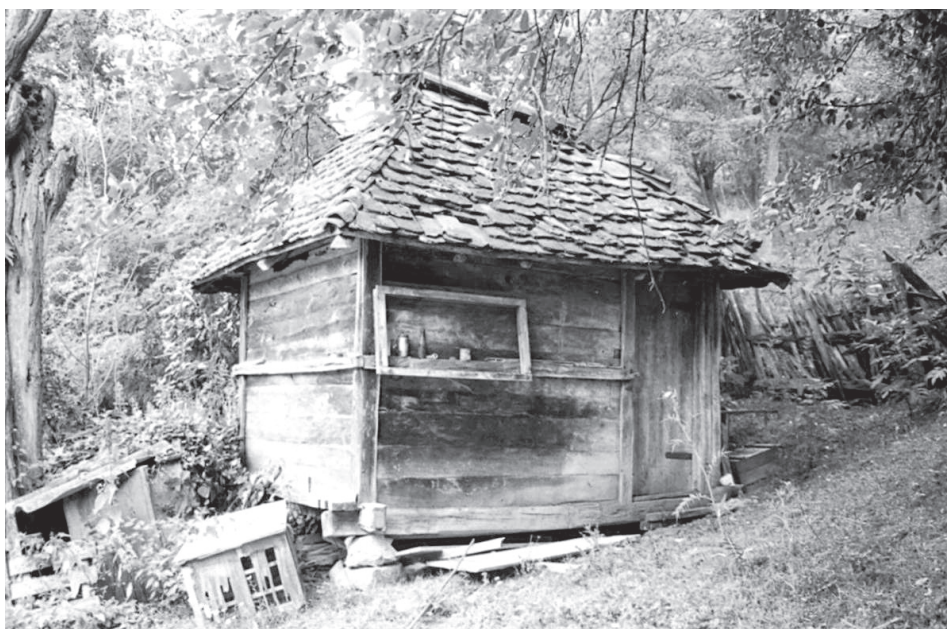
Image 14. A vajat with a frame and an infill of horizontal planks
