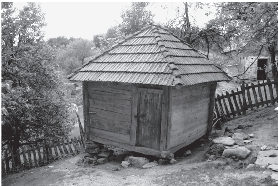
Image 7. A vajat made from thick, horizontal planks which are connected with halving joints
