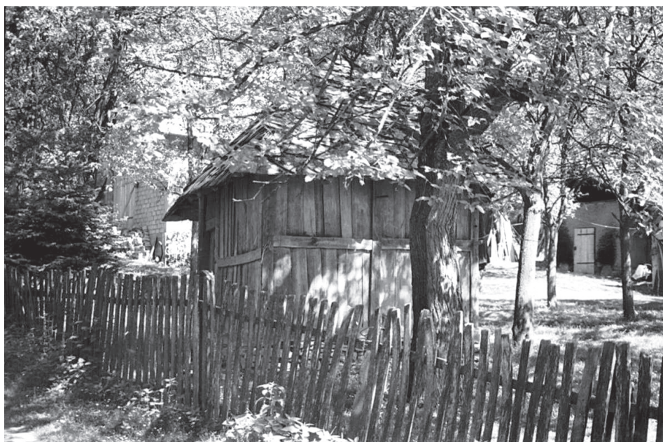
Image 19. A vajat with a frame and an infill of vertical wooden strips
