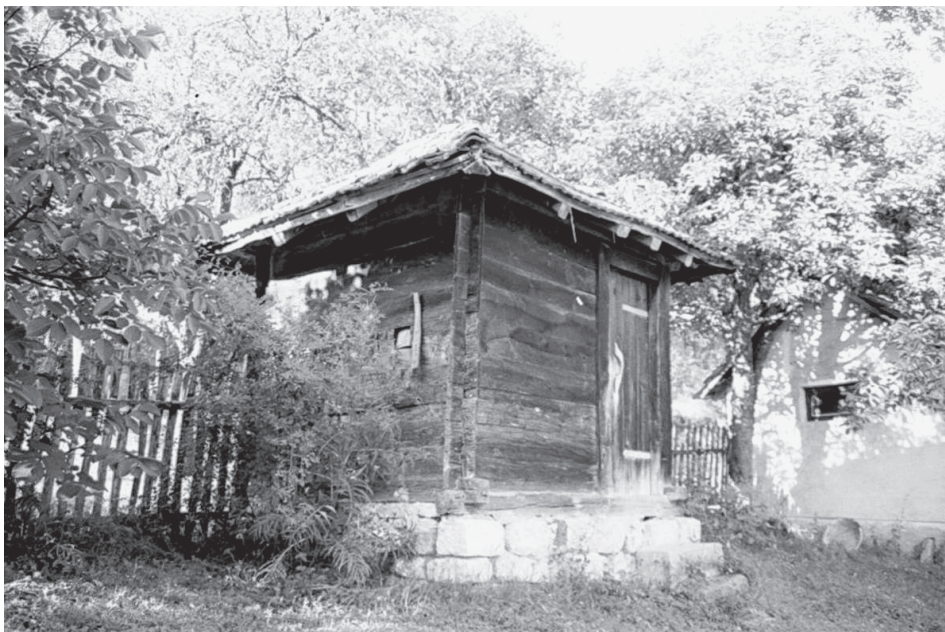
Image 2. A vajat made from thick planks which are connected with halving joints
