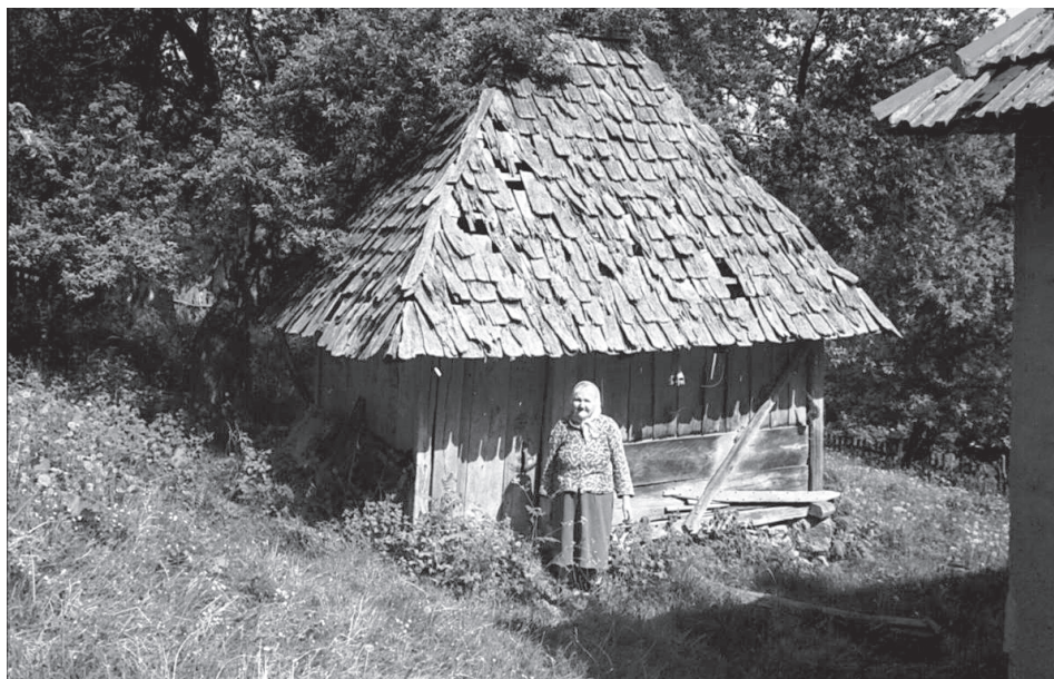
Image 17. A vajat with a frame and an infill of horizontal planks and vertical wooden strips
