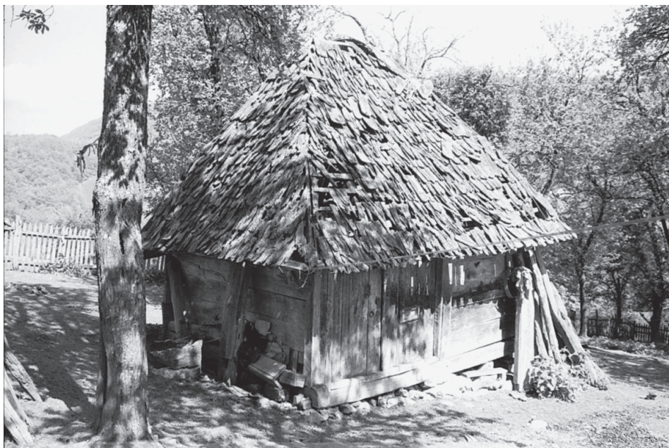
Image 9. A vajat with a frame and an infill of horizontal planks
