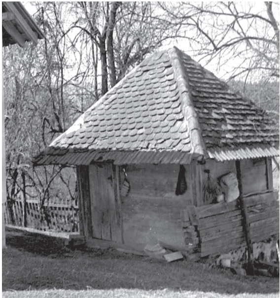
Image 15. A vajat with a frame and an infill of horizontal planks
