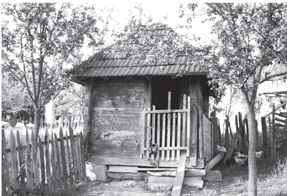
Image 3. A vajat made from thick planks which are connected with halving joints
