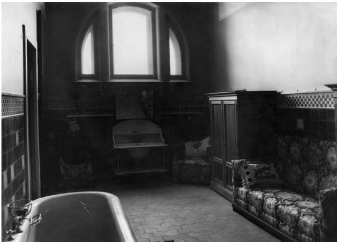
Fig. 10. Bathroom. Photograph. 1915. (Audiovisual Document Central State Archive of St. Petersburg)
