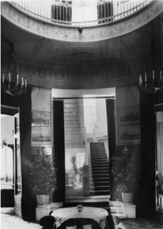
Fig. 7. Lobby. View on the main stairs. Photograph. 1915. (Audiovisual Document Central State Archive of St. Petersburg)
