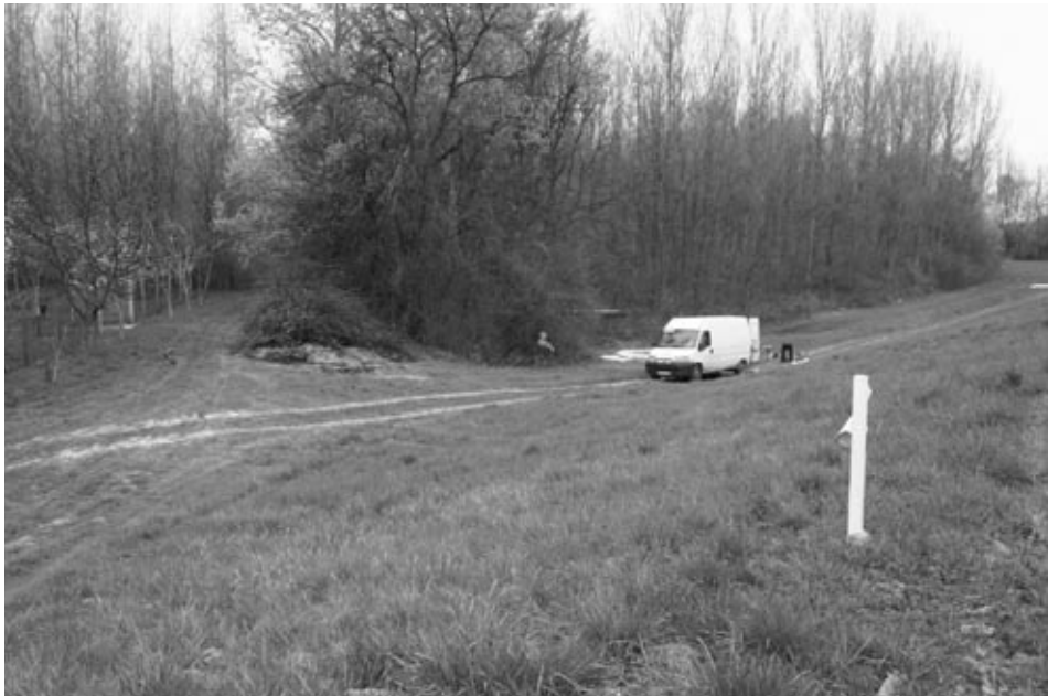
Fig. 2. – Piping (partly behind the car) at the edge of an ox-bow near Bölske (2006), with a difference in elevation of minimum two meters between ground level at the ox-bow and ground level at the adjacent high bank (Areas No. 9–10 in Tables 1 and 2)
