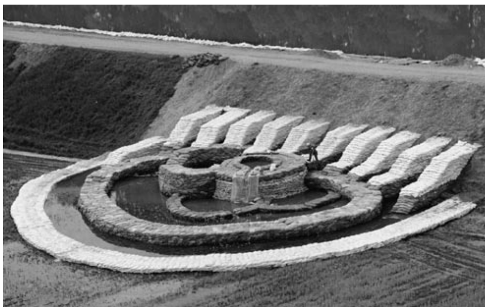
Fig. 1. – The giant piping on the Tisza's in year 2000
