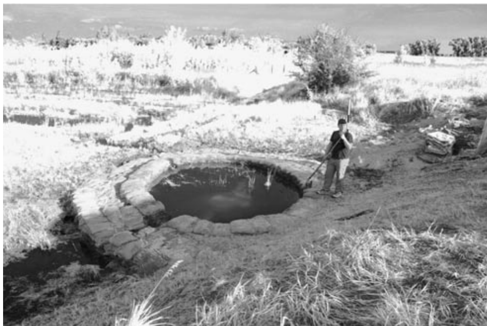
Fig. 5. – Piping at the initial section of a trench drain near Tiszaakürt in 2010 (Areas No. 19–20 in Tables 1 and 2)
