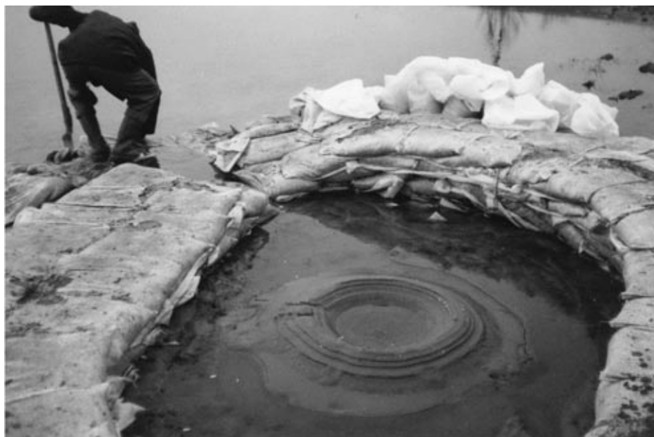
Fig. 4. – Piping at Abda (2006), some 20 m away from the dyke toe (Area No. 4 in Tables 1 and 2)
