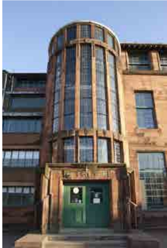
Fig. 6. East tower on northern façade
