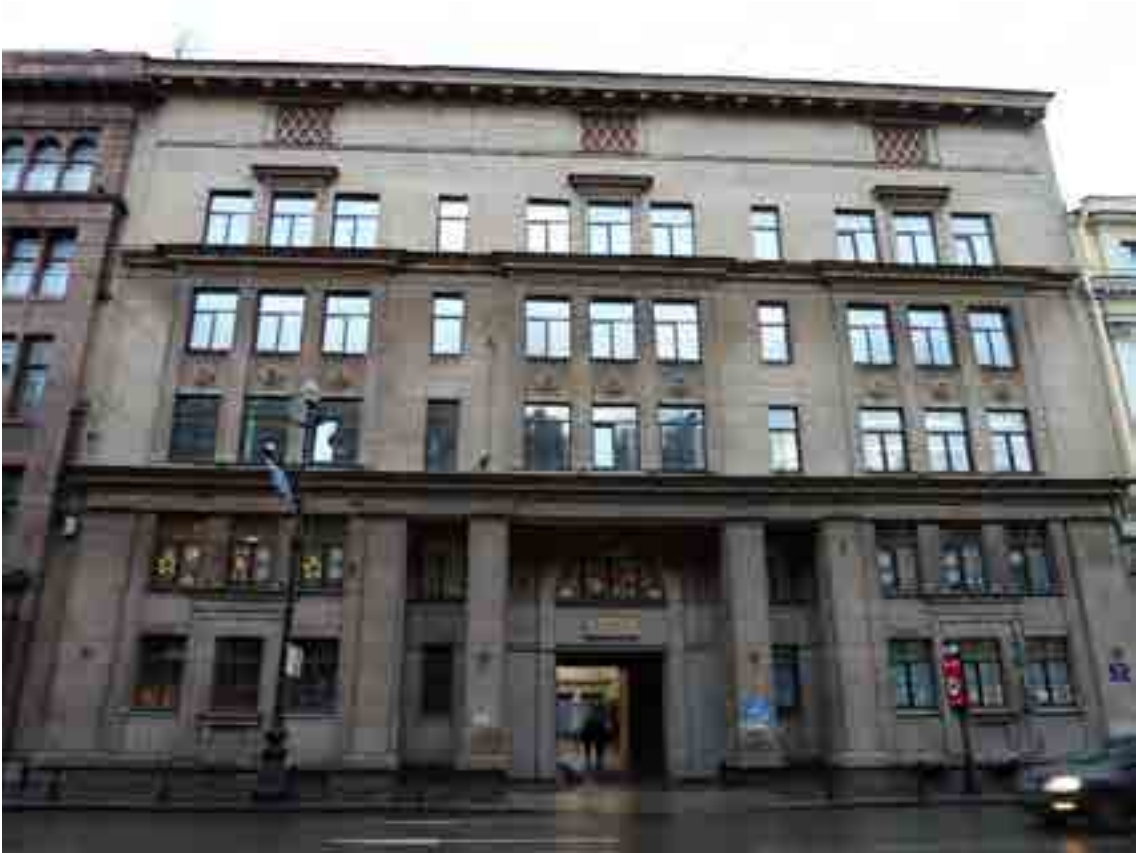
Fig. 12. School 210, Nevsky Prospekt façade
