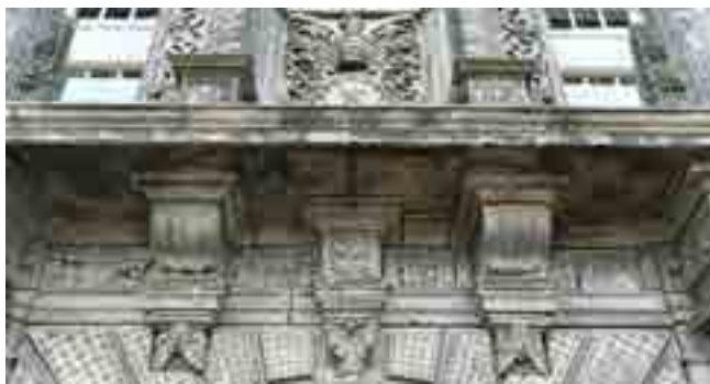
Fig. 8. George Heriot's School, Edinburgh: detail of sculptural work, north façade
