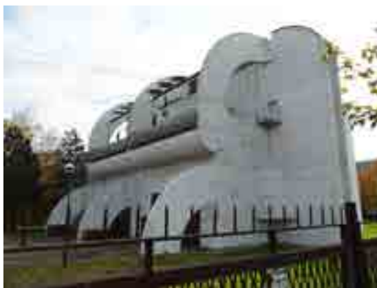
Fig. 12. Power transformer station "Filmski grad" (opposite facade)
