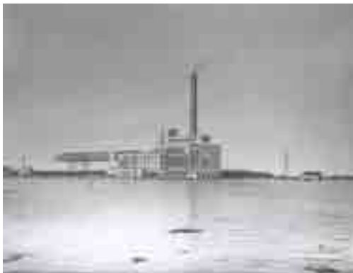
Fig. 7. Thermo-electric power plant "Strength and light", Belgrade
