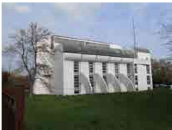
Fig. 11. Power transformer station "Filmski grad", Belgrade
