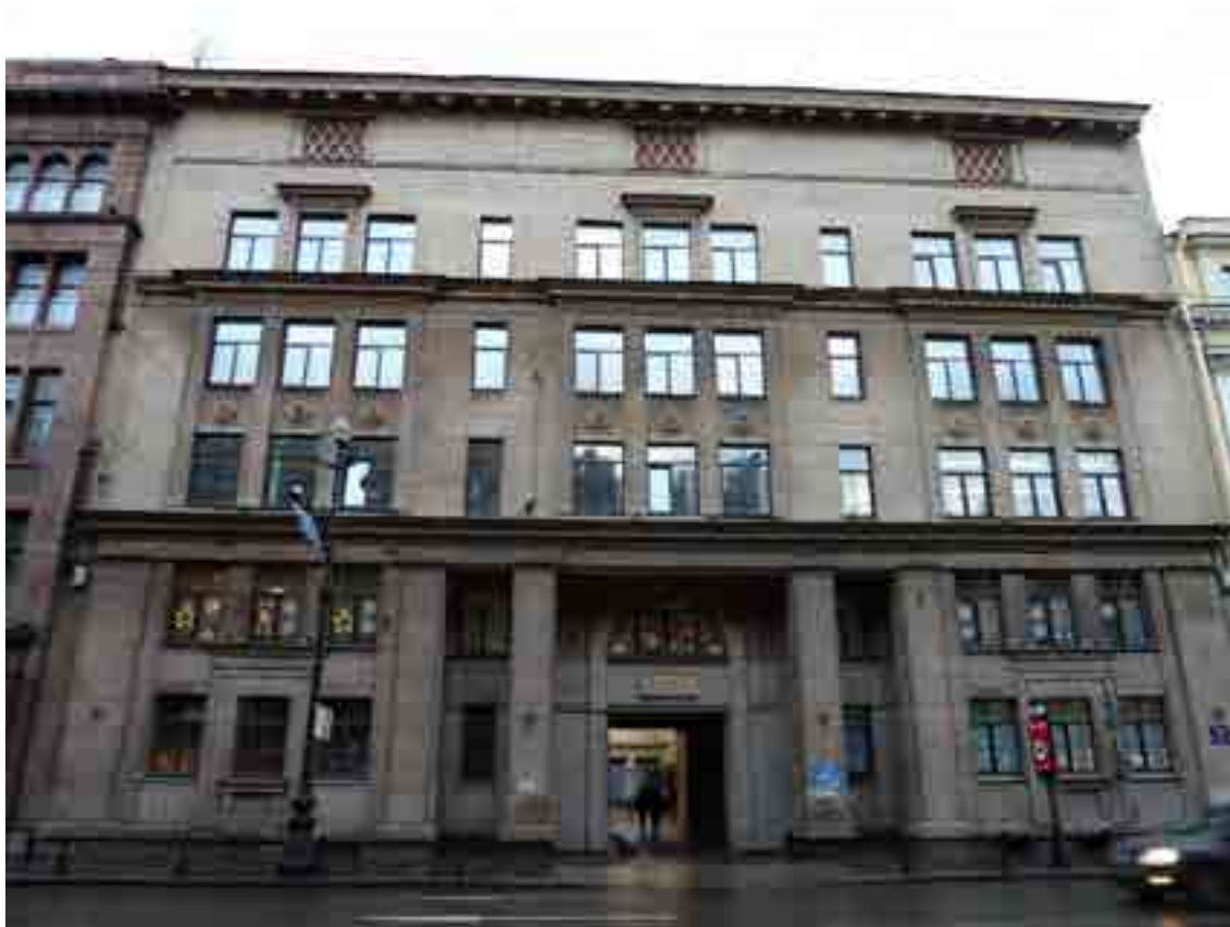
Fig. 12. School 210, Nevsky Prospekt façade
