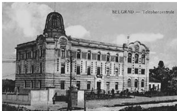
Image 8. Branko Tanazević, Main Telephone Switchboard Office (Belgrade 1908)
